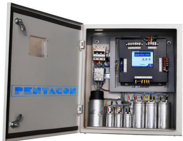
**Fig.1. Automatic Power Factor Correction (APFC)**
