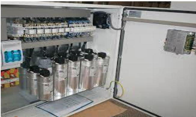
Fig -2: capacitor bank.
